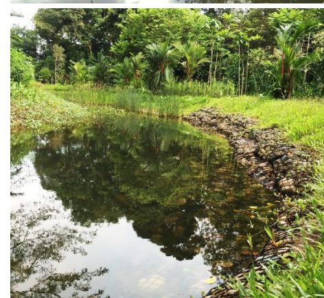
Rock chamber mattress were used as a slope stabilization method for the wetland.
