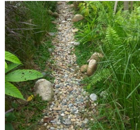
Swales installed at the site boundary
