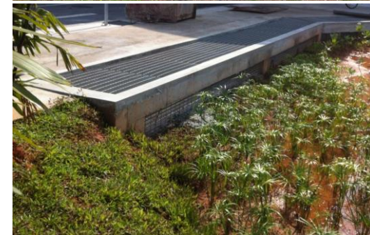
Overflow sump of the basin
